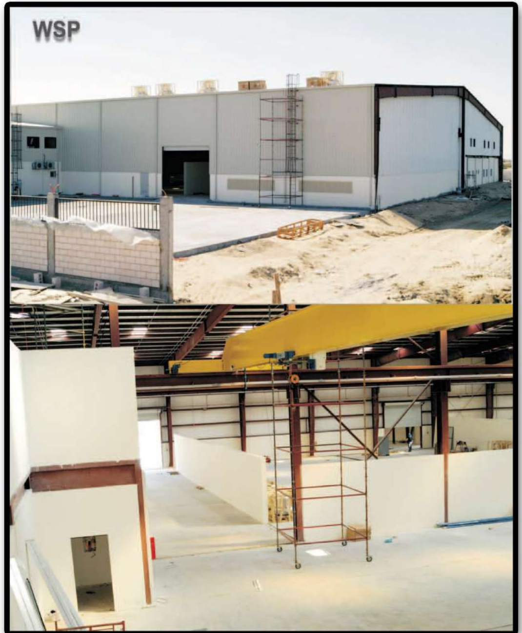
WSP PLANT EXTENSION PHASE II 2007 2nd INDUSTRIAL CITY – DAMMAM
