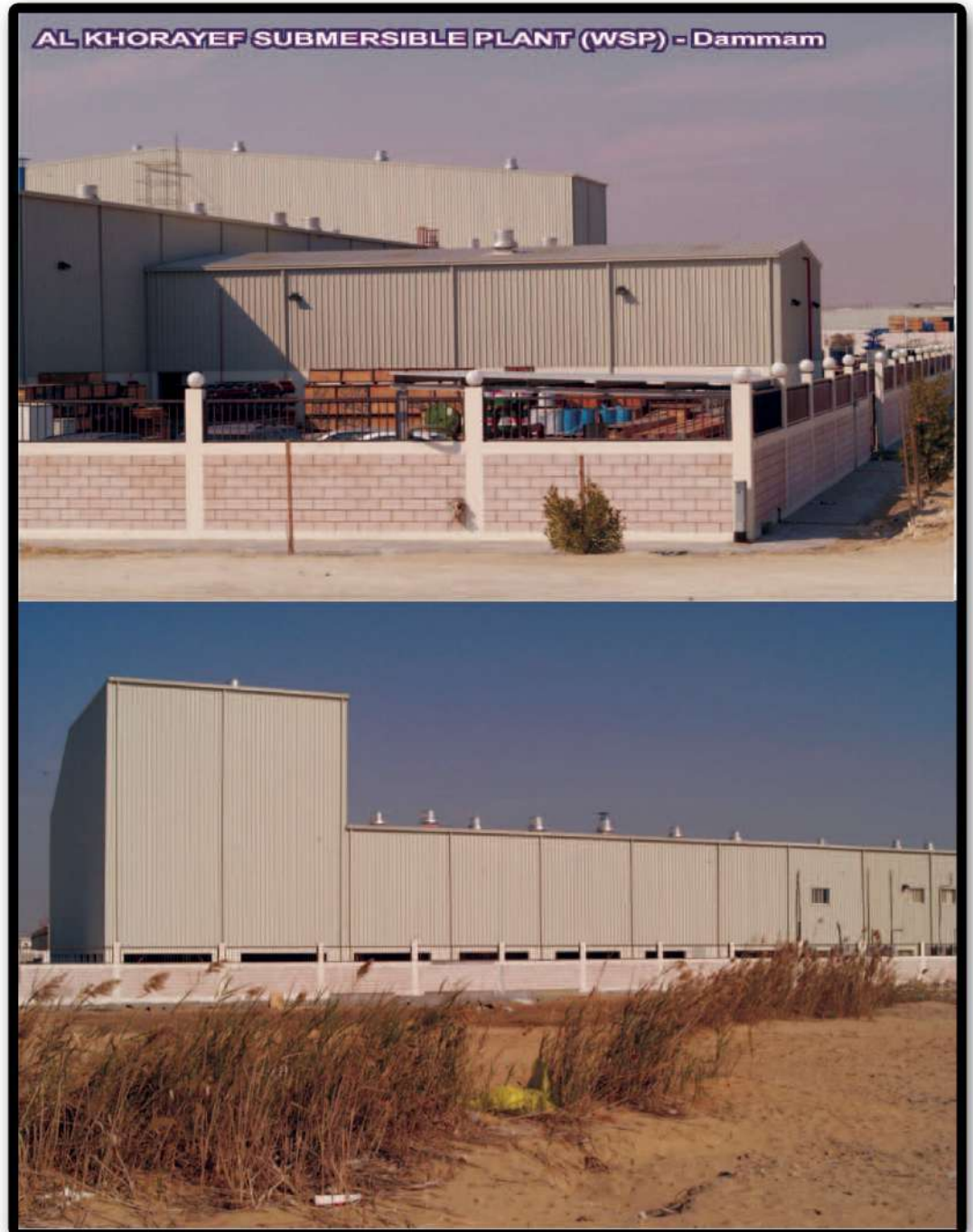
WSP PLANT & OFFICE BLDG. 2006 2nd INDUSTRIAL CITY – DAMMAM
