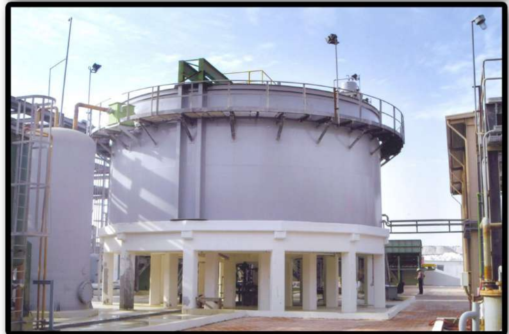
BCI NEW CHLORINE PLANT 2005 1st INDUSTRIAL CITY – DAMMAM
