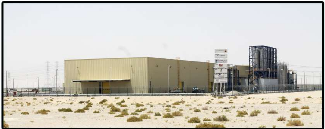
RAVAGO PRODUCTIONN & STORAGE FACILITY Al Jubail 2, KSA
