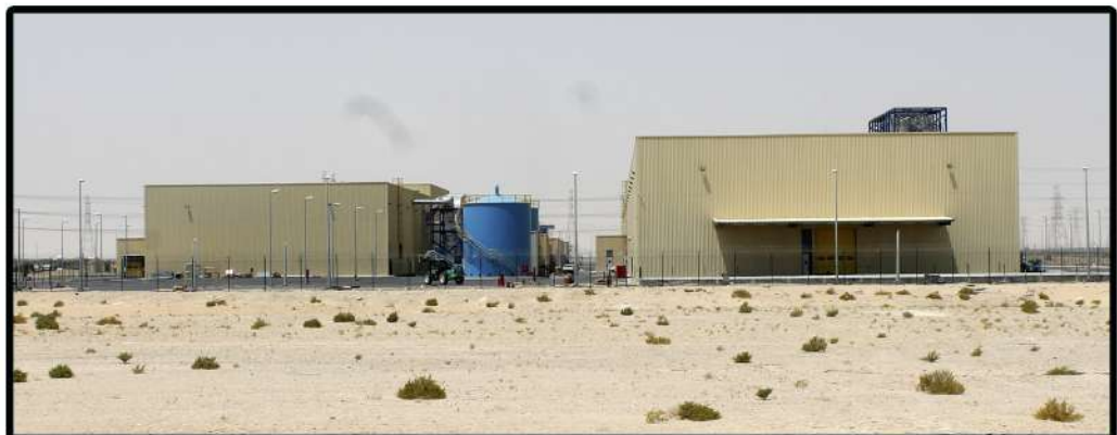
RAVAGO PRODUCTIONN & STORAGE FACILITY Al Jubail 2, KSA
