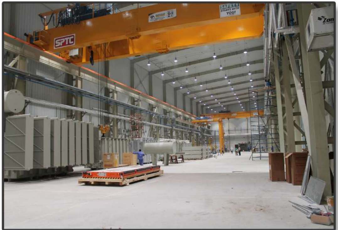
SAUDI POWER TRANSFORMERS FACTORY 2nd INDUSTRIAL CITY – DAMMAM
