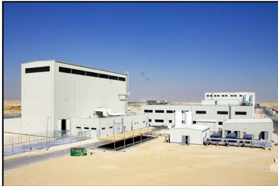
GCC-HIGH VOLTAGE LABORATORY 3rd INDUSTRIAL CITY - DAMMAM
