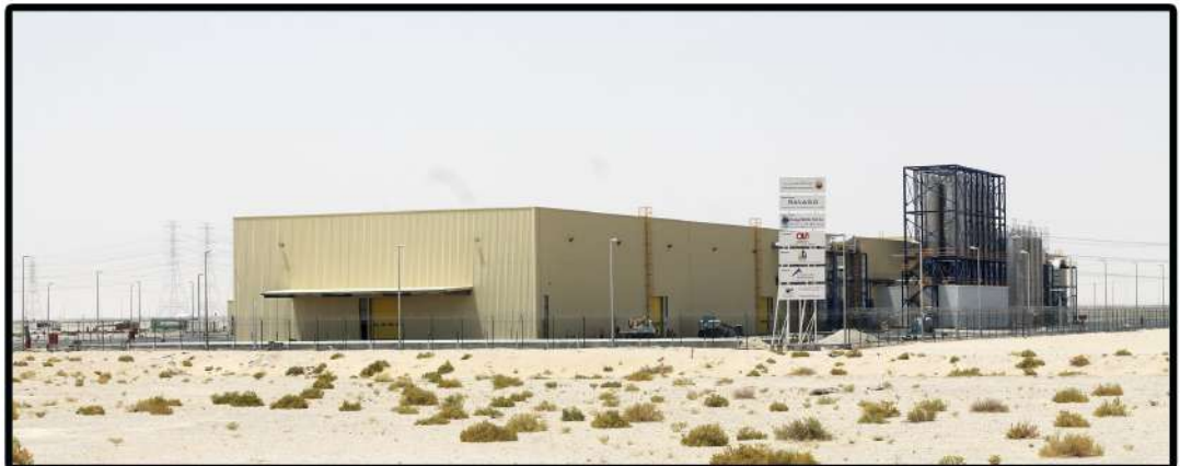
RAVAGO PRODUCTIONN & STORAGE FACILITY Al Jubail 2, KSA
