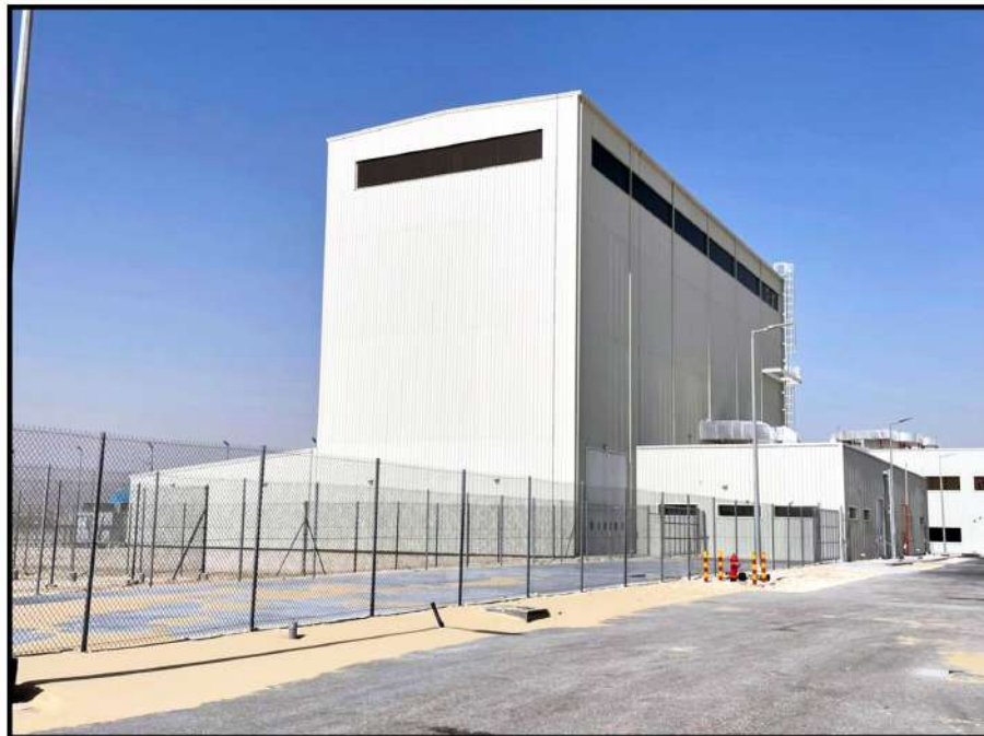
GCC-HIGH VOLTAGE LABORATORY 3rd INDUSTRIAL CITY - DAMMAM
