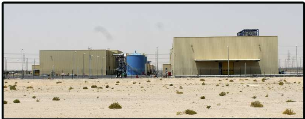
RAVAGO PRODUCTIONN & STORAGE FACILITY Al Jubail 2, KSA
