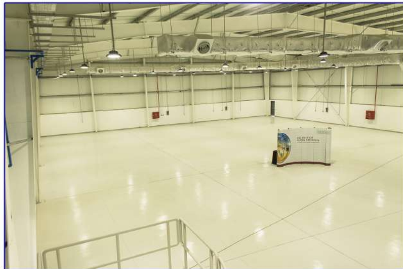
GCC- ADVANCE TESTING LABORATORY 3rd INDUSTRIAL CITY, DAMMAM KSA
