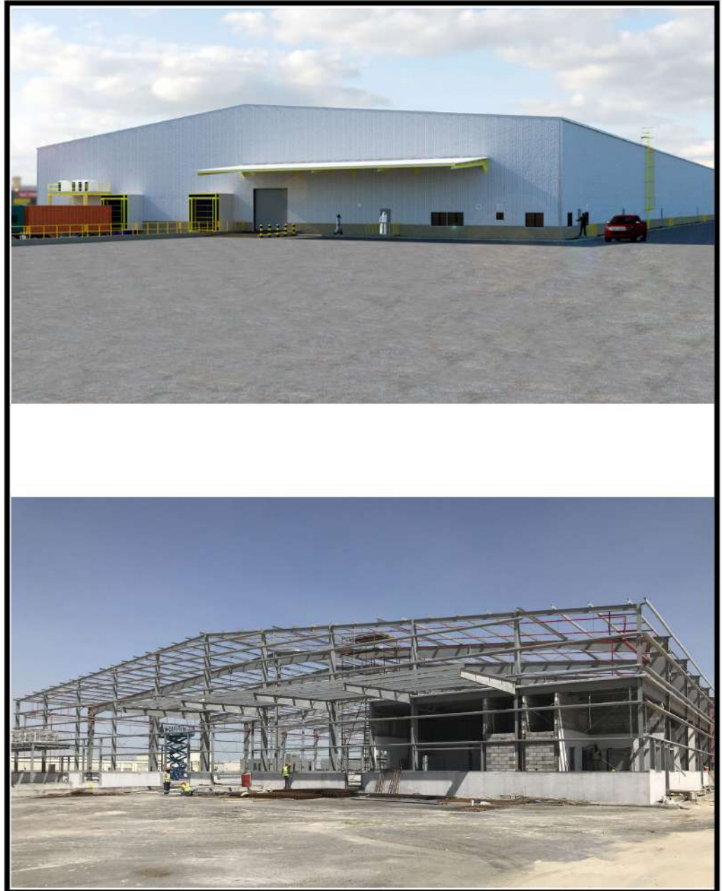
TORAY PLANT II 3rd INDUSTRIAL CITY - DAMMAM
